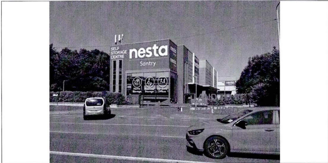
Figure 1: Photo of the only vehicular entrance to the warehousing and office facility. The only access is from the Swords Road. The Compulsory Purchase Order proposes to acquire the land at the entrance to NESTA Santry. Given the particular nature of business (customers need vehicles to deposit and collect materials), and the volume of vehicular movements associated with the operation of the business, severing the vehicular access even on a temporary basis would have a devastating impact on the business.
